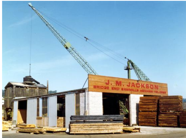
Crane provides a backdrop to new sawmill building
