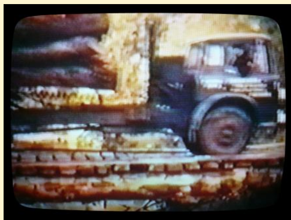
Bridge Building on the West Allen river
